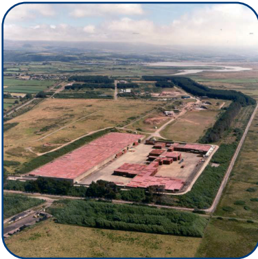
Low level waste is disposed of at a facility near Drigg in Cumbria. Image: BNFL
