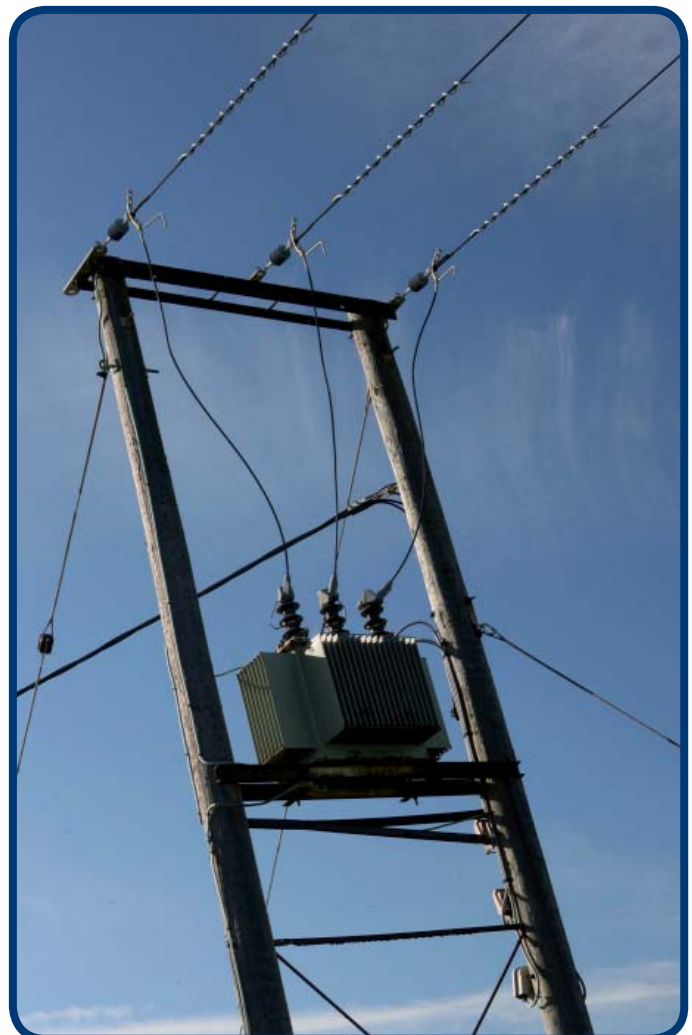
An electrical transformer
