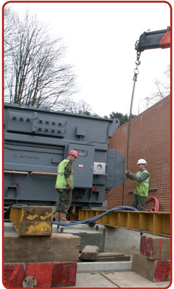
One of our transformers being installed at Maidstone, Kent
