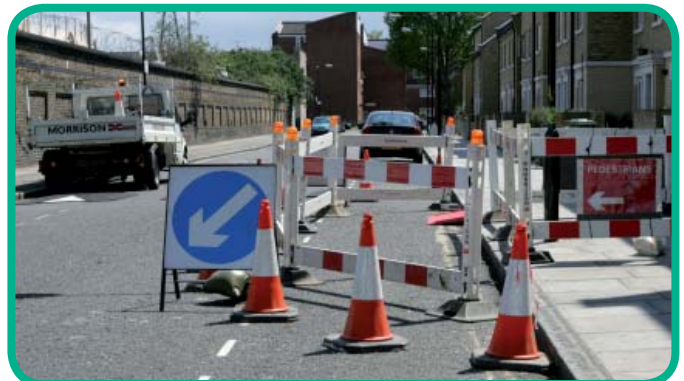
An example of our street works barriers erected to protect the public
