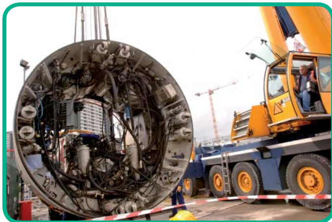
Works being undertaken to install part of one of our underground cable tunnels
