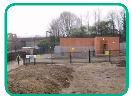
Waterside primary substation
