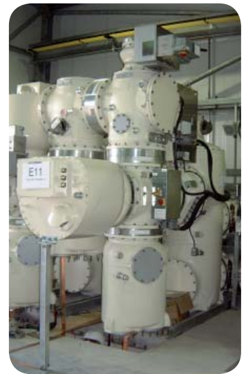
132kV substation with equipment filled with SF 6
