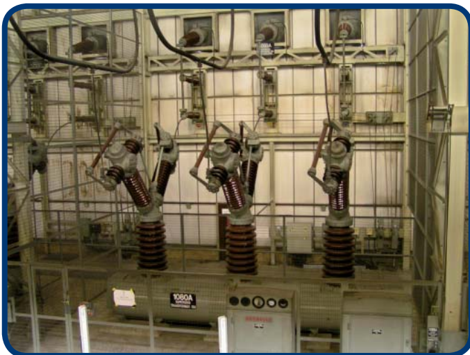
A supergrid that forms part of our network
