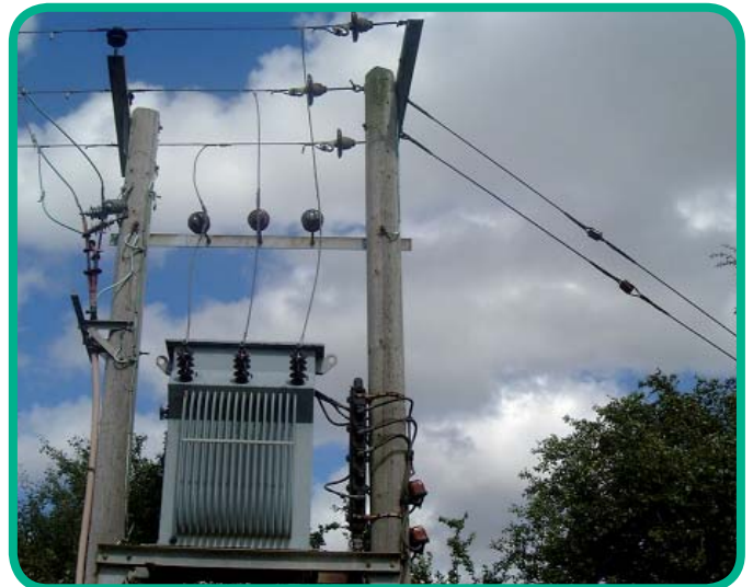
An overhead transformer, one of our many network assets
